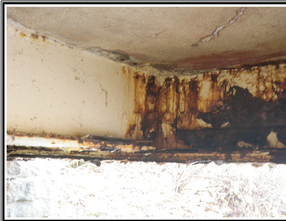
FLOORBEAM 10 & RIGHT GIRDER CONNECTION Fracture Critical Detail
