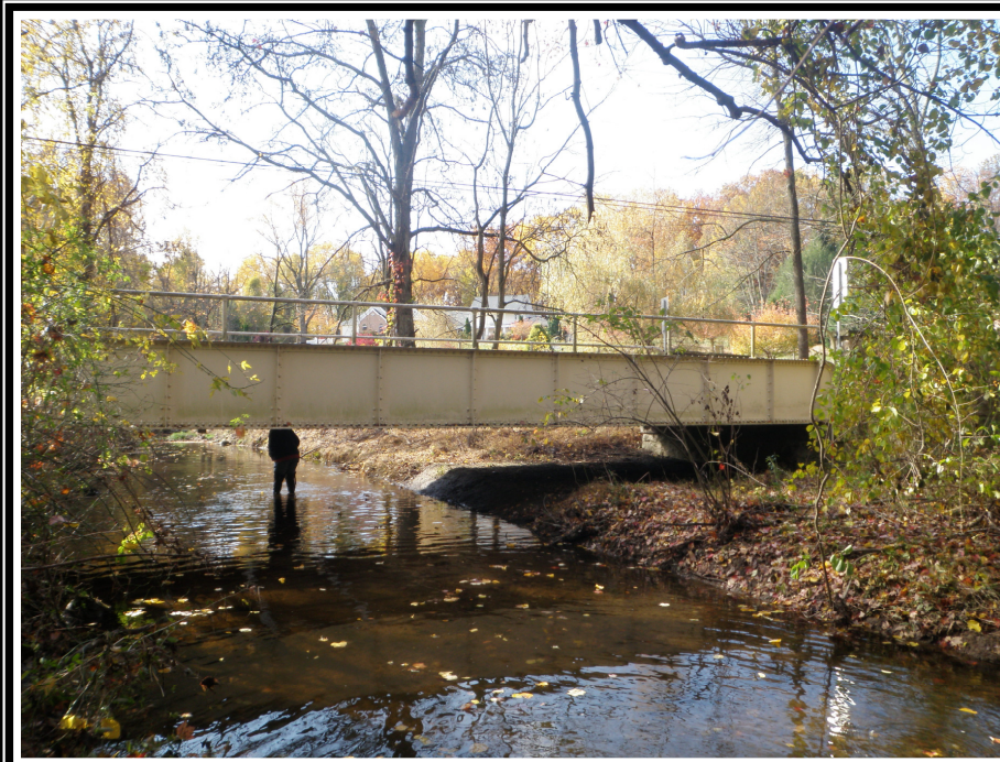
UPSTREAM (LEFT) ELEVATION North
