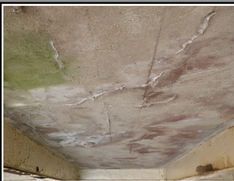
DECK UNDERSIDE, BAY 9 Looking Upstream
