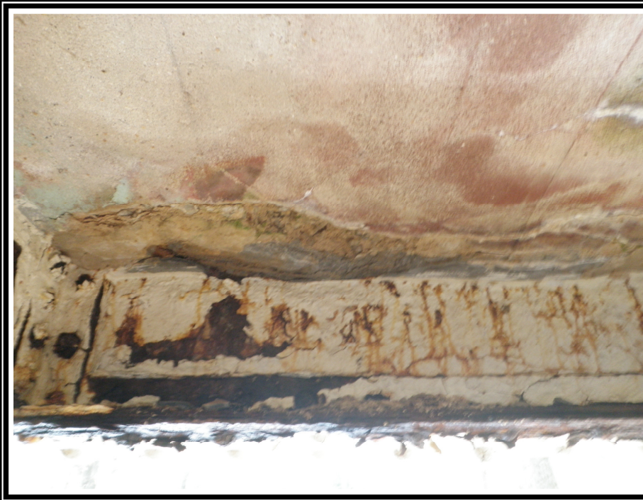
DECK UNDERSIDE, BAY 6 Right Girder, Looking Downstream
