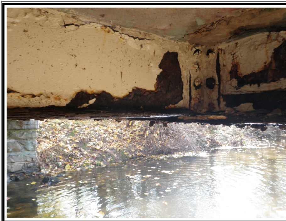
FLOORBEAM 7 & RIGHT GIRDER CONNECTION Looking Downstream
